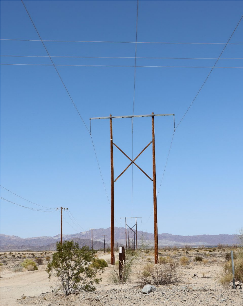
Photograph 3. Existing wooden H-frame (56 to 74 feet tall)
