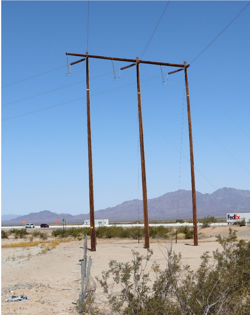
Photograph 1. Existing wooden three-pole structure (56 to 80 feet tall)
